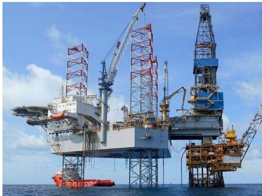
Tom Prosser jack-up drilling rig (© Noble Corporation)
