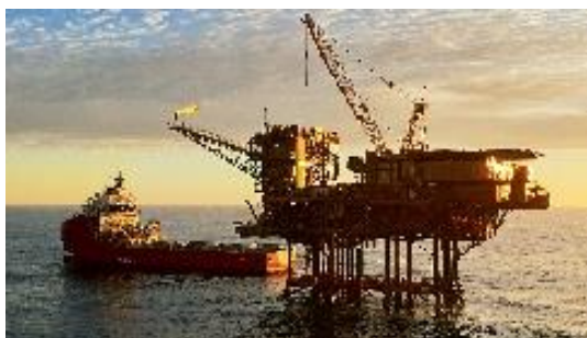
The MMA Leeuwin survey vessel alongside the Barracouta platform
