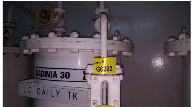
Photo 68 G6292 3rd Deck Engine Room, Gardina 30 Oil Tank Top Bracket Flange, Sight Glass – Gasket (Chrysotile)
