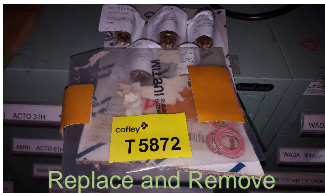
Photo 134 T5872 F Deck - No.2 Equipment Room, Drawer DB4 - Gasket Loose, Boil Off Valve Bulkhead penetration insulation Gland (Orange) (Chrysotile)
