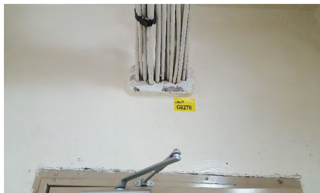
Photo 122 G6276 A Deck - Waste Storage Room, Bulkhead Above Entrance Door - Gasket (Chrysotile)
