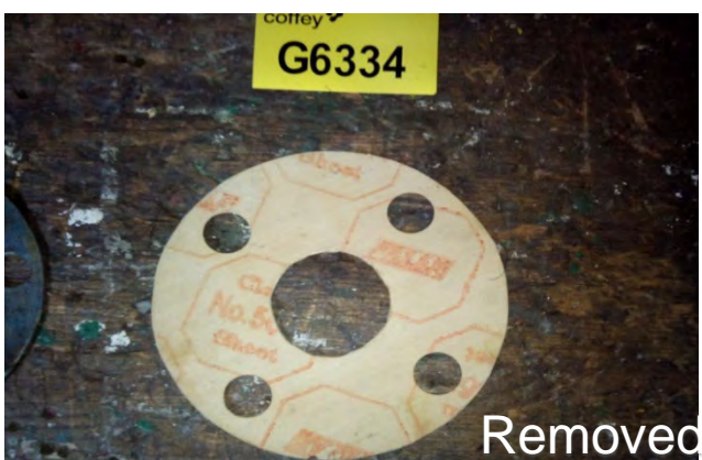
Photo 99 G6334 Upper Deck - External, Deck Workshop - Gasket Loose 'Pillar No. 5611' (Presumed Positive)(Chrysotile)
