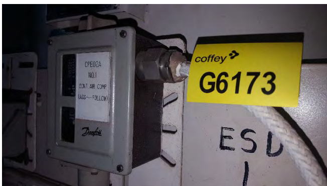
Photo 13 G6173 4 th Deck - Engine Room, FWD Port, Control Air Receiver, Pressure Transmitter Conduit – Putty (Chrysotile)
