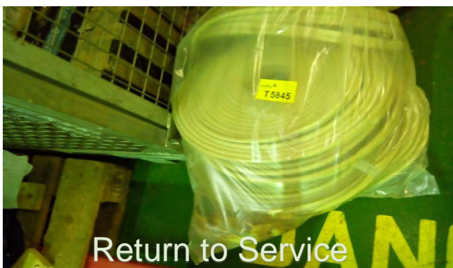
Photo 143 T5845 2nd Deck Storage Area, Contained for Reassurance, Return to Area Above Cabinets 'BF' & 'BE'– Boiler Lagging 680.01.01.G14 (No Asbestos Detected)
