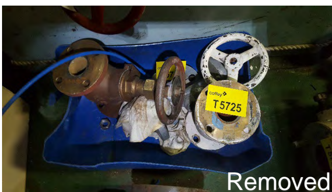
Photo 27 T5725 3rd Deck Workshop Mezzanine, Starboard, Fore, Adjacent Handrail, Stored Items (In Blue Plastic Tub) – Gasket (UMF)
