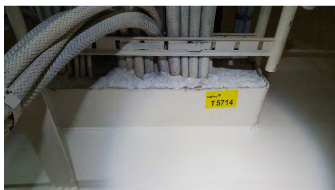
Photo 20 G6187 4 th Deck Purifier Room, Under Lube Oil No.1 Purifier Control Cabinet, Conduit – Putty (Chrysotile)
