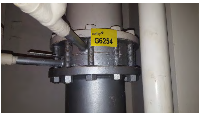
Photo 59 G6254 3rd Deck Engine Room, Port Gas Hood, Gas/Inlet Flange – Gasket (UMF)
