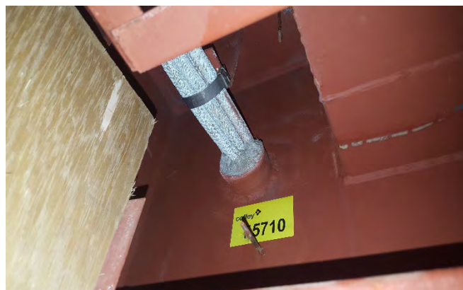
Photo 128 T5710 B Deck - Sauna, Conduit Penetrations (Throughout) – Bulkhead penetration insulation (Chrysotile)
