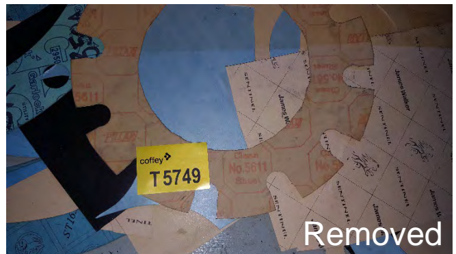
Photo 36 T5749 3rd Deck - Workshop, Bulkhead penetration insulation Draws, First Draw (Labelled Off-Cuts) - Gasket 'Pillar Clean Sheet No. 5611' (Orange Font, Beige Back) (Presumed Positive)
