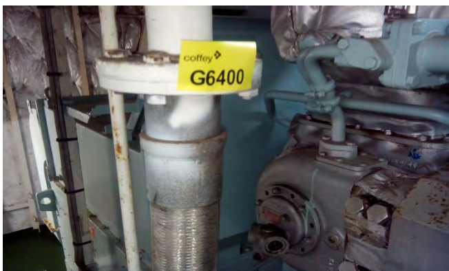
Photo 121 G6400 Upper Deck - Emergency Generator Room, Sump Vent, Flexible Hose Flange – Gasket (UMF)
