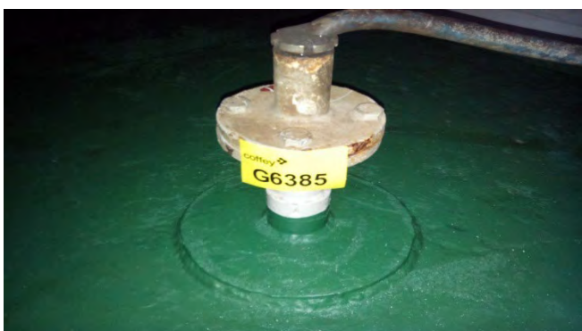
Photo 119 G6385 Upper Deck Pipe Passage Starboard, Transducer Adjacent 45 WBT – Gasket (UMF)
