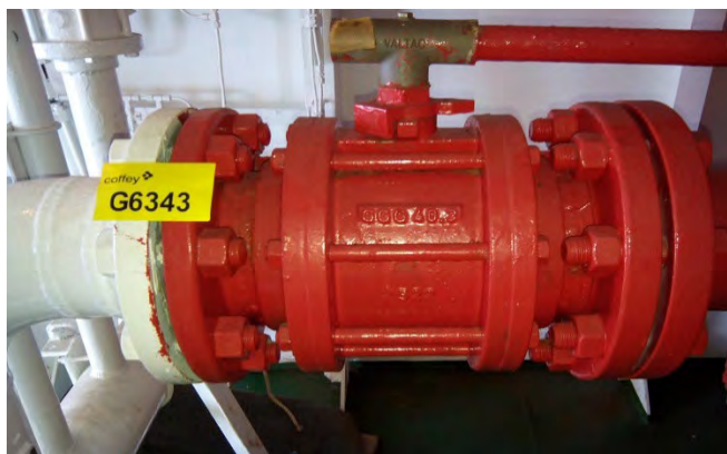
Photo 103 G6343 Upper Deck - Dry Chemical Unit Room, Aft, Outlet Storage, Under Manifold – Gasket (Chrysotile)
