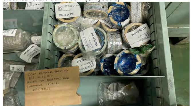
Photo 206 ZA9300 Stores - BF1, Soot blower packing - Port 639.10.01.018 (Chrysotile)
