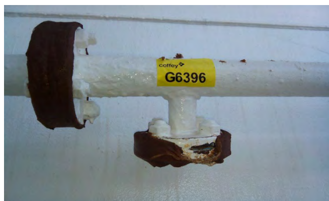
Photo 130 G6396 C Deck - External, Port Stairs, Deluge System, Flange Joint-Gasket (UMF)
