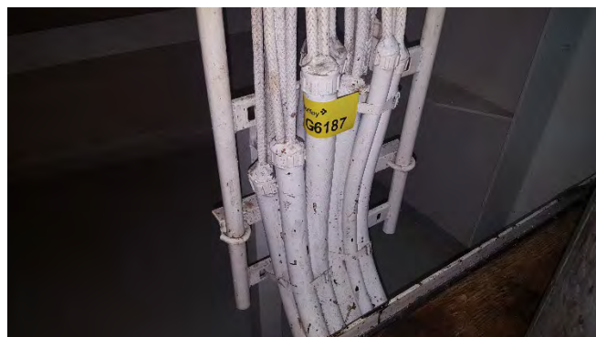
Photo 20 G6187 4 th Deck Purifier Room, Under Lube Oil No.1 Purifier Control Cabinet, Conduit – Putty (Chrysotile)
