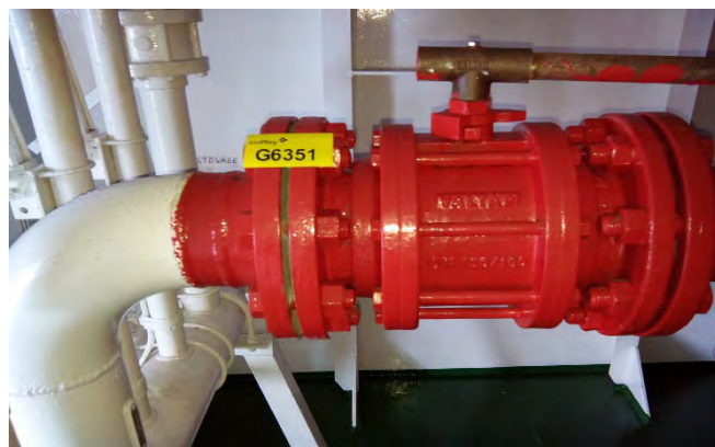
Photo 104 G6351 Upper Deck - Dry Chemical Unit Locker, Under Manifold - Gasket (Chrysotile)
