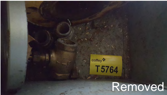
Photo 31 T5764 3rd Deck - Workshop Mezzanine, Starboard, Fore, Adjacent Handrail, Stored Items (Light Blue Metal Box – Debris (Chrysotile)
