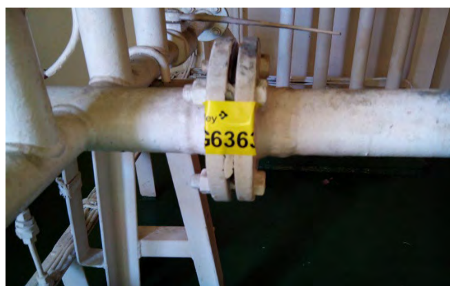
Photo 104 G6351 Upper Deck - Dry Chemical Unit Locker, Under Manifold - Gasket (Chrysotile)
