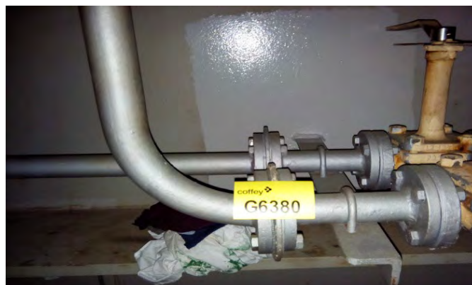
Photo 116 G6380 Upper Deck Pipe Passage Starboard, Valve to Sampling Line) - Gasket (UMF)
