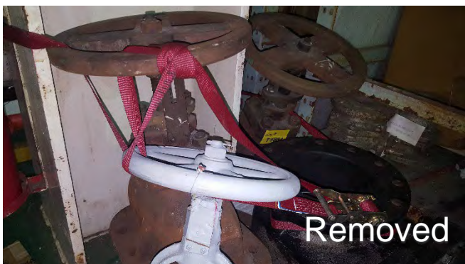
Photo 85 T5864 2nd Deck - Storage Area, Structural Column Adjacent 2nd Shelf from Fore – Gasket to Bonnet of x 2 Valves (Rusting) (Chrysotile)
