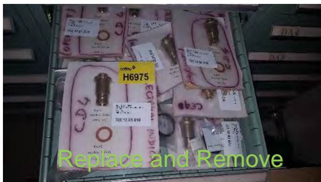
Photo 147 H6975 F Deck, No.2 Equipment Room, F3 DB4 722.12.01.G10 Boil Off Gas Valves, Gasket (Pink Backing Black Cursive Font) (Chrysotile)
