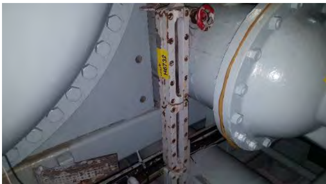
Photo 67 H6732 2nd Deck, IGG Room, Sight Glass Level, Gasket (Chrysotile)
