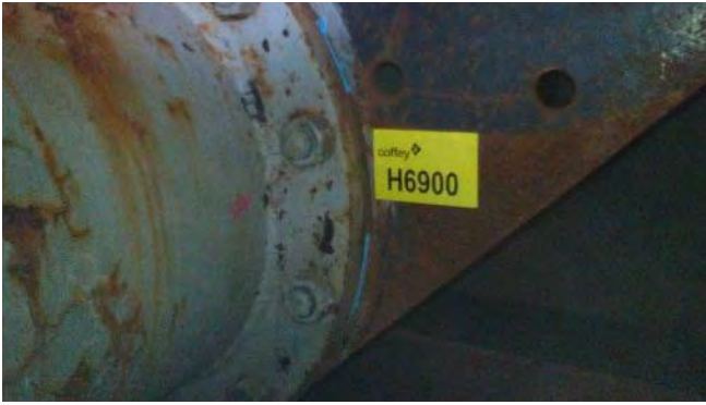
Photo 127 H6900 Upper Deck, Port Passage, Spectacle Piece Port Frame 65, Gasket (UMF)
