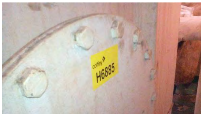
Photo 122 H6885 Upper Deck, Cargo Motor Room, Gas Vent Drain, Tank Manhole, Gasket (Chrysotile)
