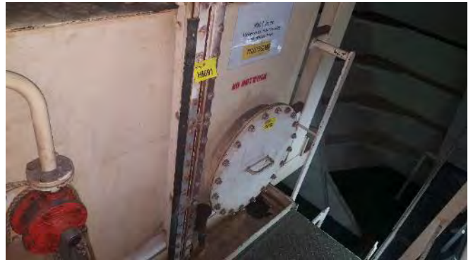
Photo 54 G6691 3rd Deck, Steering Flat, Storage Tank S2V68 Sight Level Glass, Gasket (Chrysotile)
