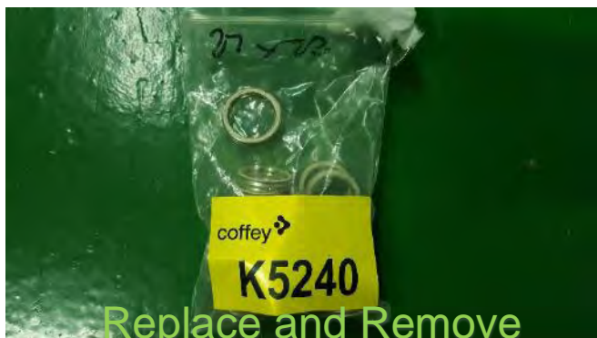
Photo 157 K5240 2nd Deck, 2SA, BF2 Boiler Gauge Glass, Gasket (Metal) (Chrysotile)
