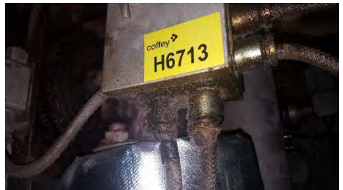
Photo 60 H6713 3rd Deck, Burner Tops, Starboard Boiler Conduit No.5 Soot Blower Junction Box, Putty (Chrysotile)
