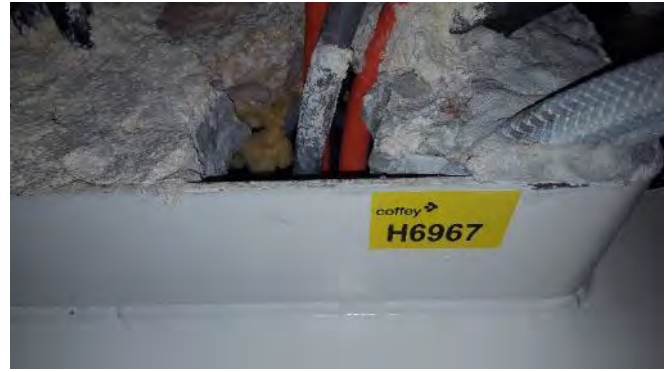
Photo 140 H6967 F Deck, Electric Cable Space, Inboard Deck Head, Packing (Chrysotile)
