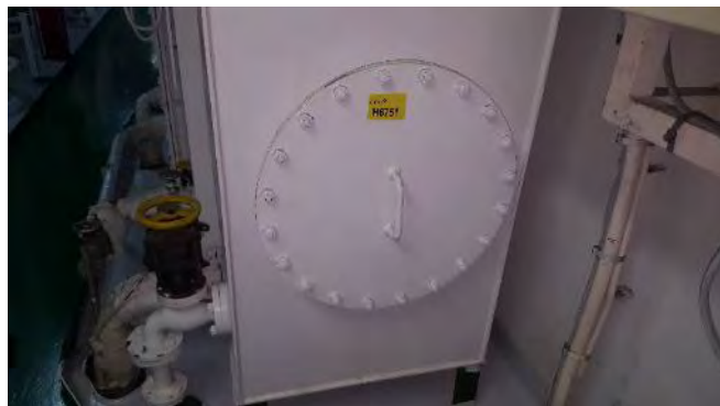
Photo 74 H6751 2nd Deck, Starboard, L.O. Renovation Tank (Small) Manhole, Gasket (Chrysotile)
