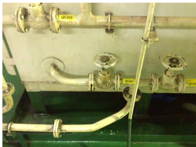
Photo 40 Q5367 Focsle store -starboard Aft - hyd oil store tk outlet Gasket to hyd oil store tk outlet port
