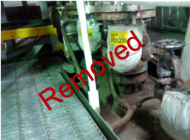
Photo 57 FD5239 2nd Deck, Engine Room, No.2 Boiler Drum Safety Valve, Aft, Woven Rope (Chrysotile)
