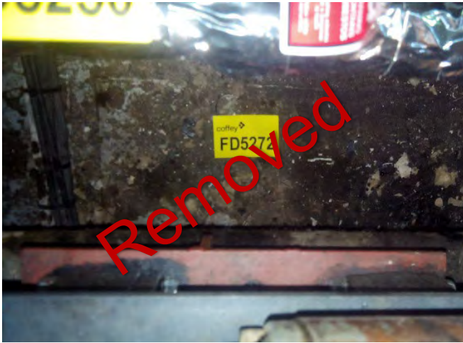
Photo 53 FD5272 4th Deck, Engine Room, Boiler No.2 Top, Mixed Debris (Chrysotile)
