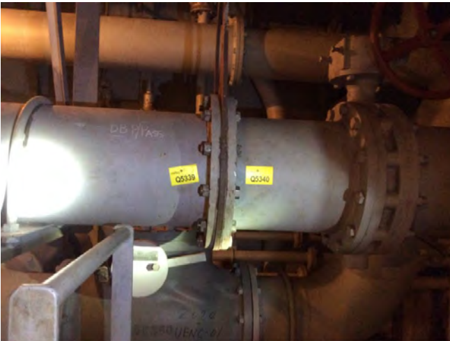
Photo 43 Q5339 Port UDPP- IG 2 Dbpp Spectacle piece downstream Gasket
