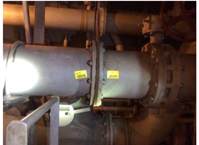
Photo 44 Q5340 Port UDPP Spectacle piece up stream Gasket
