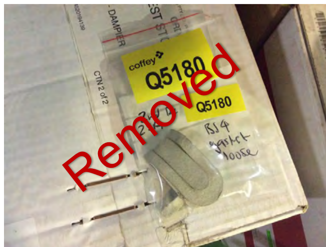
Photo 22 Q5180 2nd deck - 2sa - bj4 drawer Loose sight Gasket - no markings
