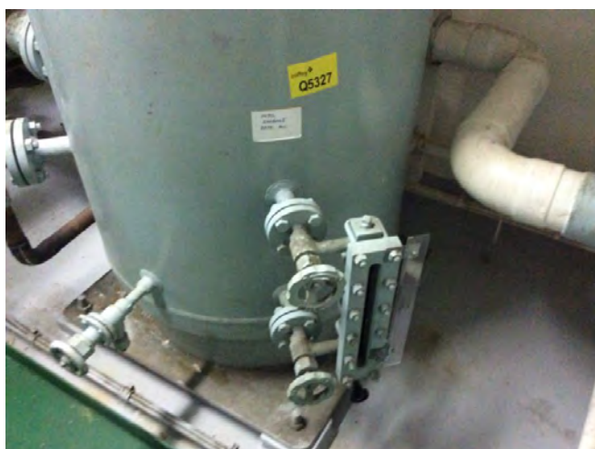
Photo 15 Q5327 2nd deck - starboard fwd - main a/c oil receiver Sight glass gasket
