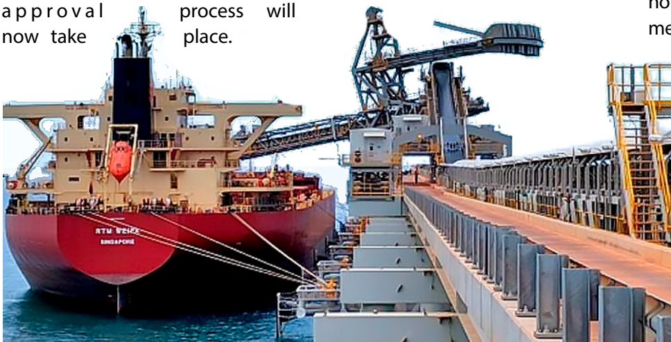
First bauxite from Amrun was shipped from Yarwun alumina refinert in December 2018. image courtesy Rio
