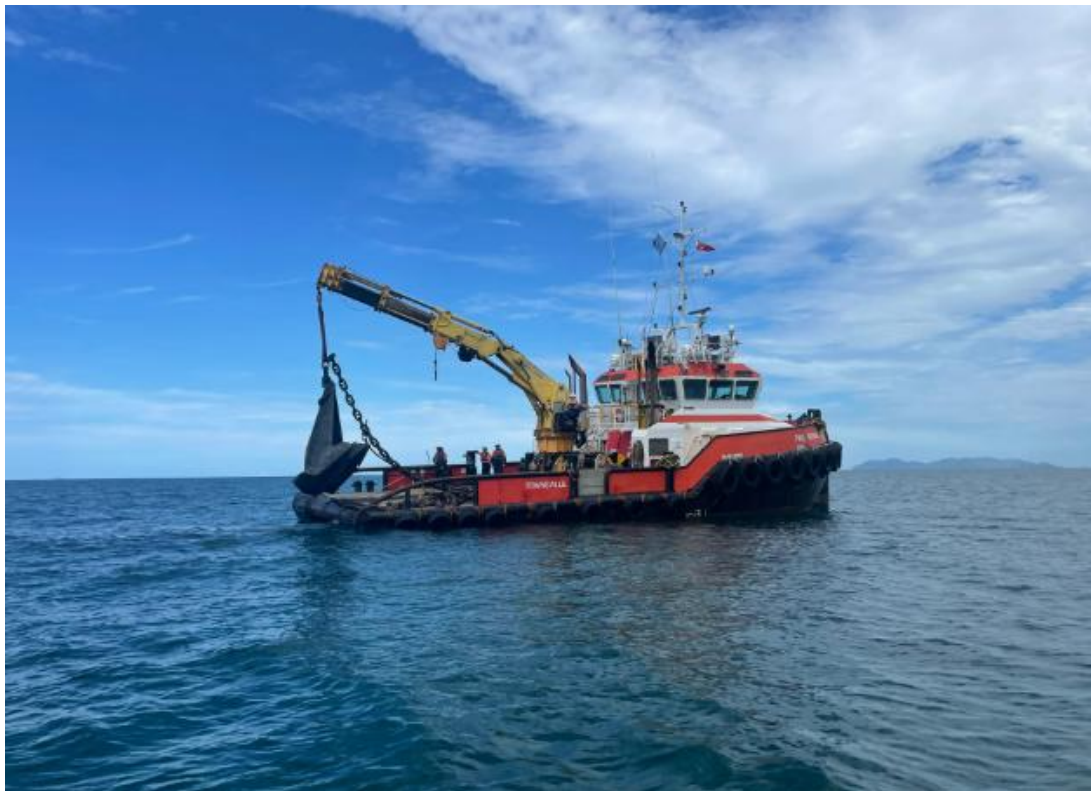
Image: Pacific Marine Group: Installation of a cyclone mooring:
